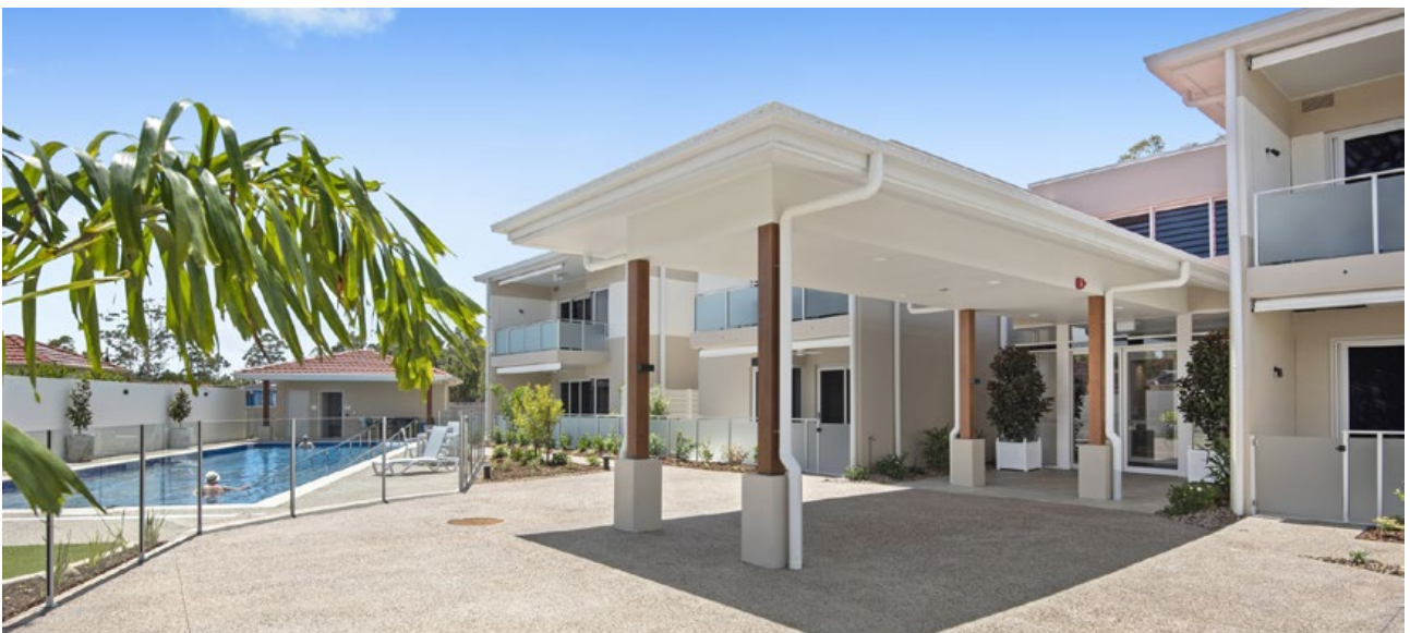
Block B Apartment construction is well underway, with two-thirds of the 34 apartments already sold!
